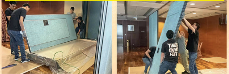
Repairs and refurbishment of floors and replacement of defective operable partitions for the Braidwood's Hall 布雷活堂修理和翻新地板，以及更換損壞的屏風
